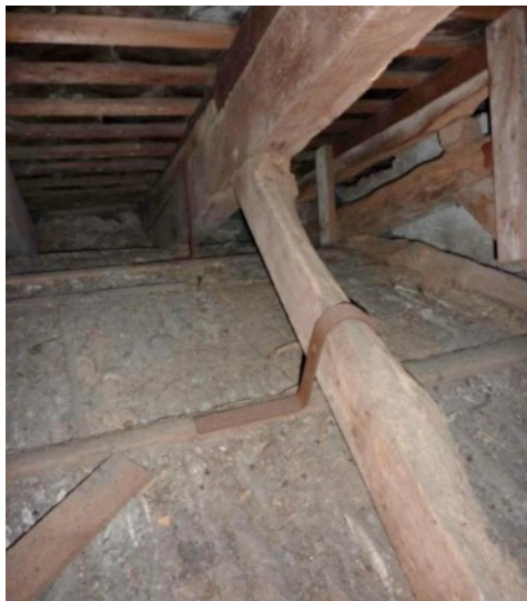
Timbers in the roof void
