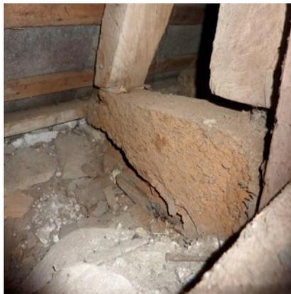
Beetle damage to arch brace and tie on north side of the Nave
